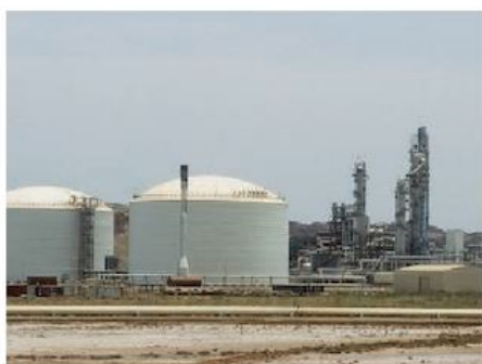
A chemical plant for making ammonia
