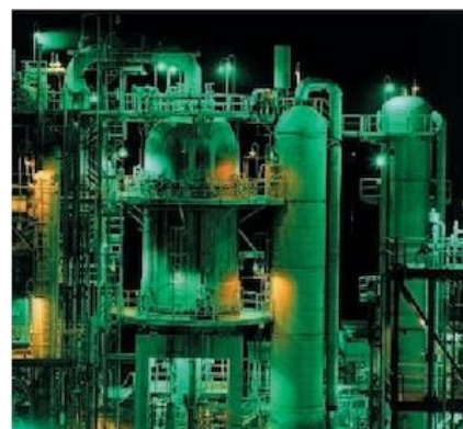
A cat cracker like this one is used to split long-chain hydrocarbons into shorter-chain hydrocarbons and alkenes
