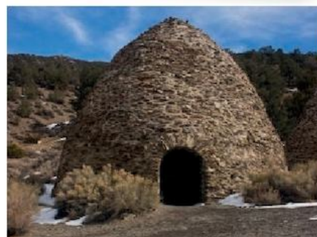
Charcoal kilns like these have been used for centuries to provide the carbon for metal extraction
